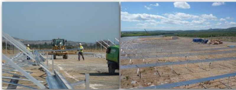
Installation des structures
